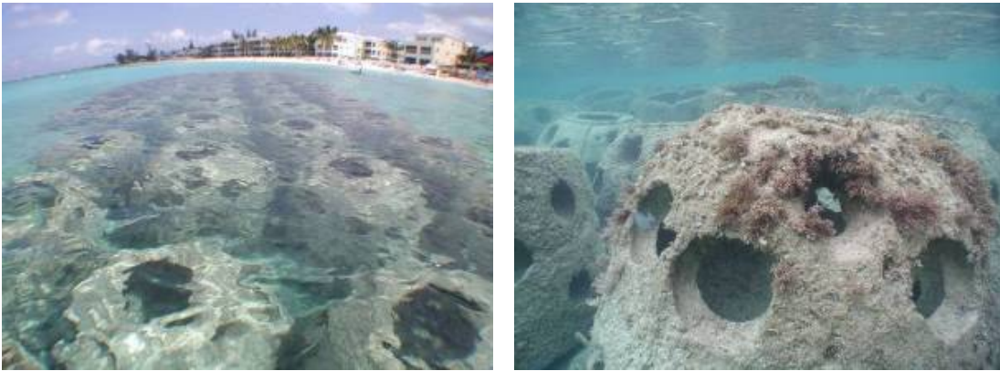
Figure 13. Above and Underwater Photographs of the Reef Ball Breakwater Submerged Breakwater offshore of the Grand Cayman Marriott Beach Resort
