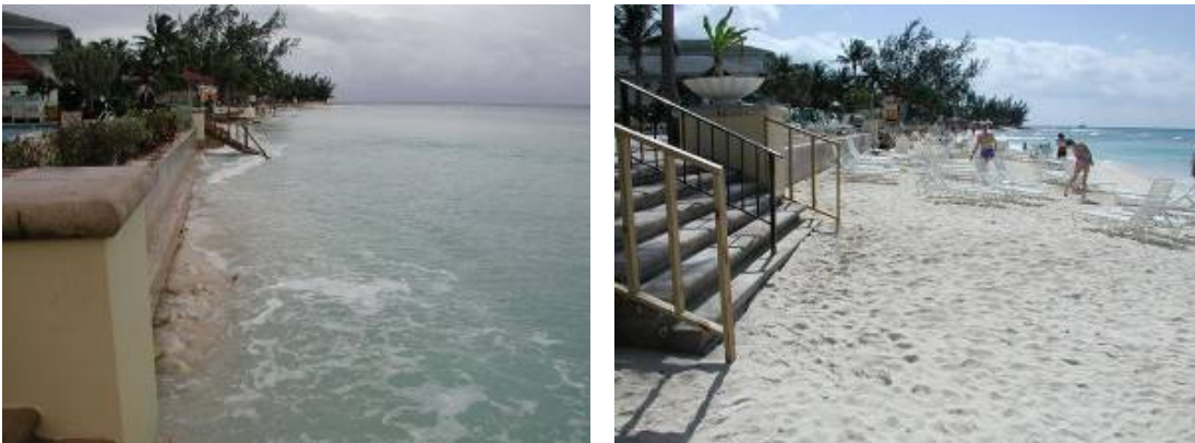
Figure 14. Marriott Beach Before and After Reef Ball Breakwater Installation Photo from Fall 2002 (L) and February 2003 (R) after the breakwater installation
